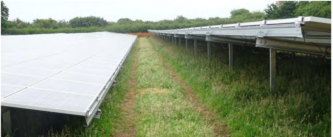
Photo 16: After Panels Bolted-on
