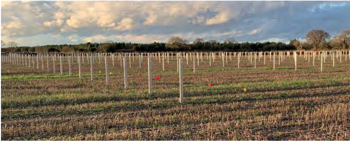
Photo 15: Legs Being Installed (this at Tiln Farm, Retford, in Janaury 2023)
