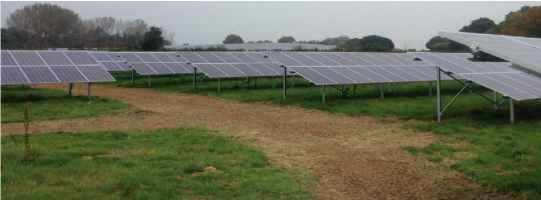
Photo 20: An Example of Track Restoration
