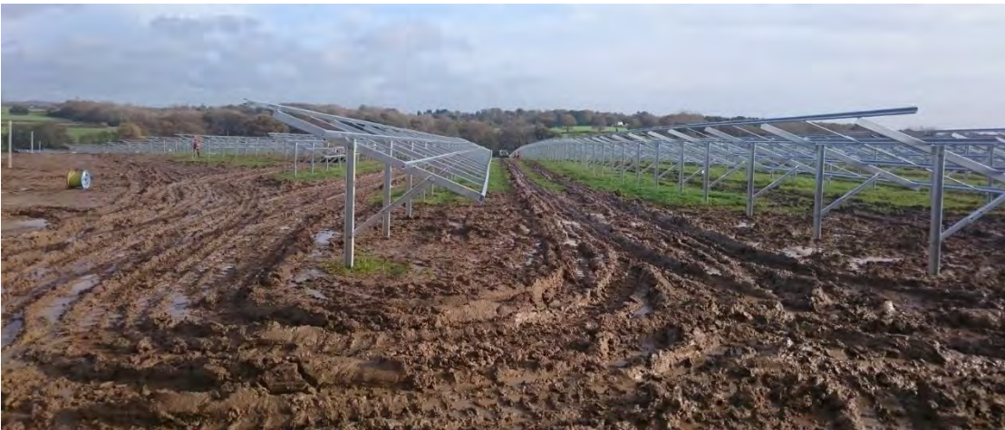
Photo 18: An Example of Winter Installation Affecting Soils
