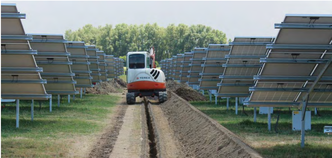
Photo 17: Trenching Works
