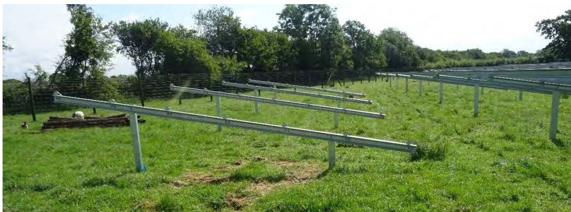
Photo 14: Legs Installed (this at Bentham Farm, Purton, Summer 2015)
