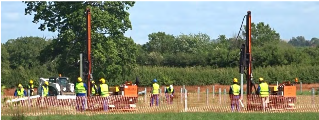
Photo 13: Legs Being Installed
