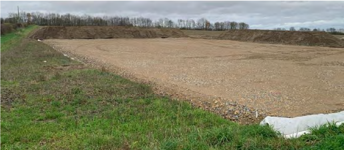
Photo 22: Example of Construction Compound
