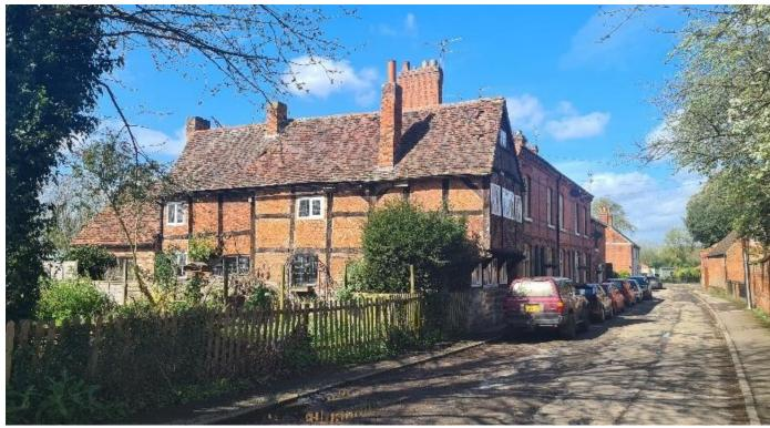
Figure 59 - Mid C17 house with C18 and C19 alterations. Timber framed with red brick nogging, in the main herringbone (Zone 1)
