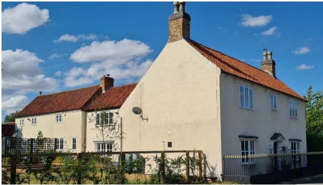
Figure 32 - Ivy House Farm (Main Road)
