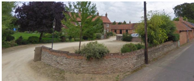
Figure 18 - Yew Tree Farmhouse Garden Wall with Partial Rubble Plinth
