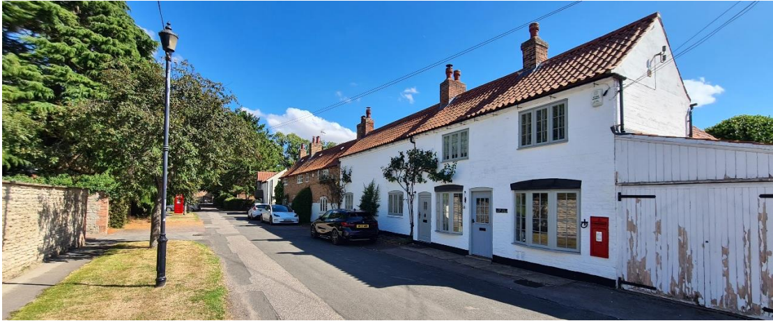
Figure 12 – Town Street towards Hawksworth Manor
