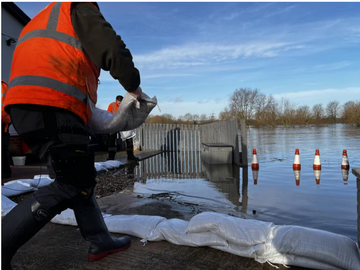
Officers work to contain flooding
