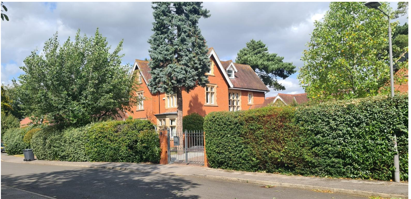
Figure 32 – The Professor's House - A Victorian red brick dwelling, with gables emphasised by the over sailing roof and timber bargeboards. The ashlar mullioned and transomed sash windows contribute to the building's significance.
