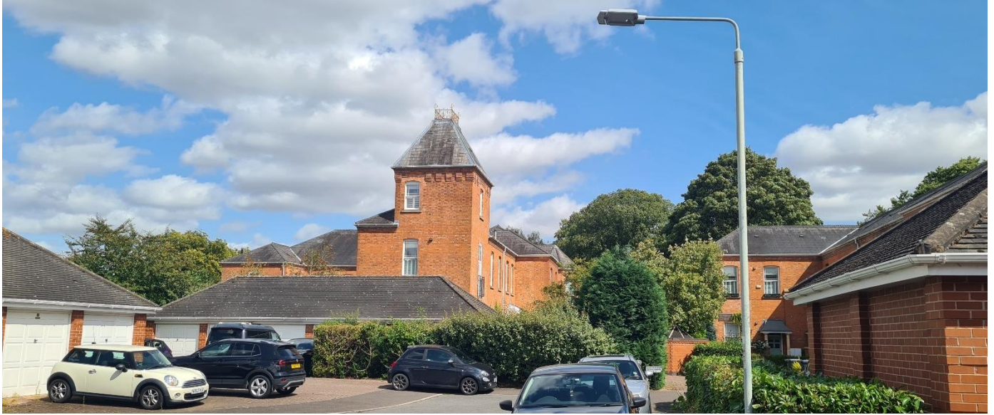
Figure 31 - One of the four towers found on the ward buildings. These have pyramidal state roofs with wrought iron finials and brick eaves detailing.
