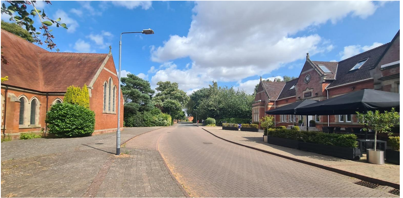
Figure 9 - standing opposite one another the chapel and administration building mark the key focal point of the Conservation Area
