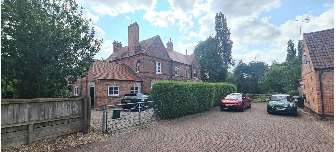
Figure 33 - Home Farmhouse is constructed of a darker coloured brick to the other Victorian buildings within the conservation area. It has arched brick lintels, an ashlar door surround, brick string courses and a plain tile roof.
