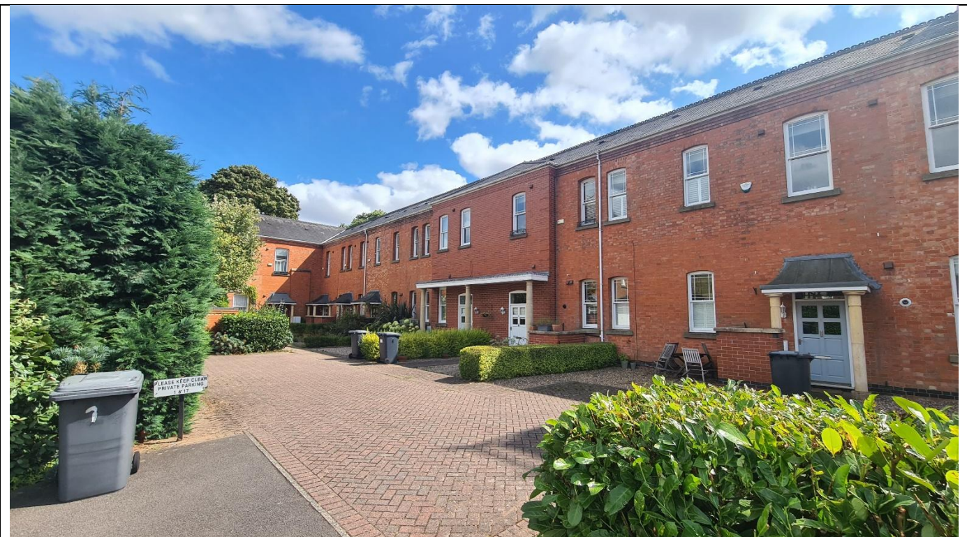
Figure 25 - Hard landscaping consists of asphalt highways. The block paving denotes more private area.
