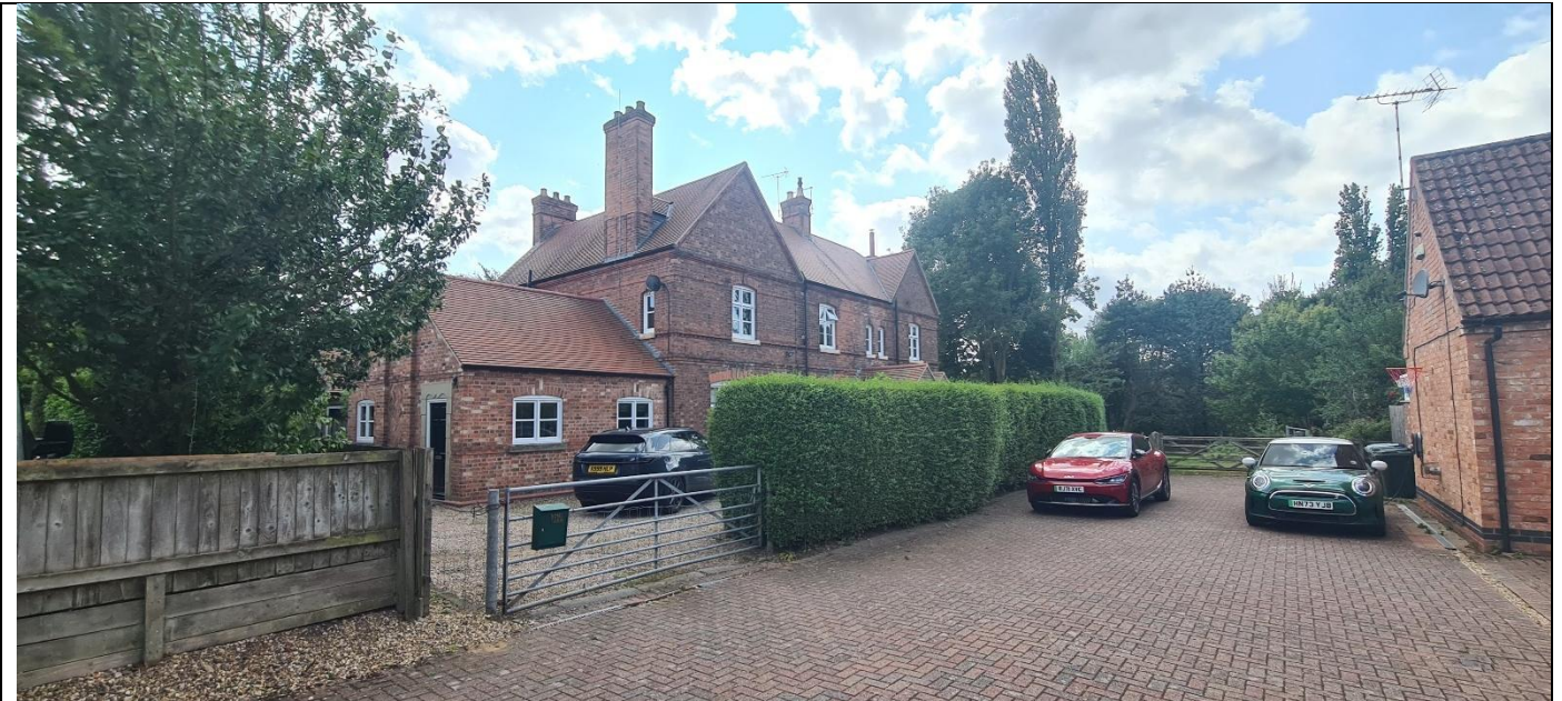
Figure 33 - Home Farmhouse is constructed of a darker coloured brick to the other Victorian buildings within the conservation area. It has arched brick lintels, an ashlar door surround, brick string courses and a plain tile roof.
