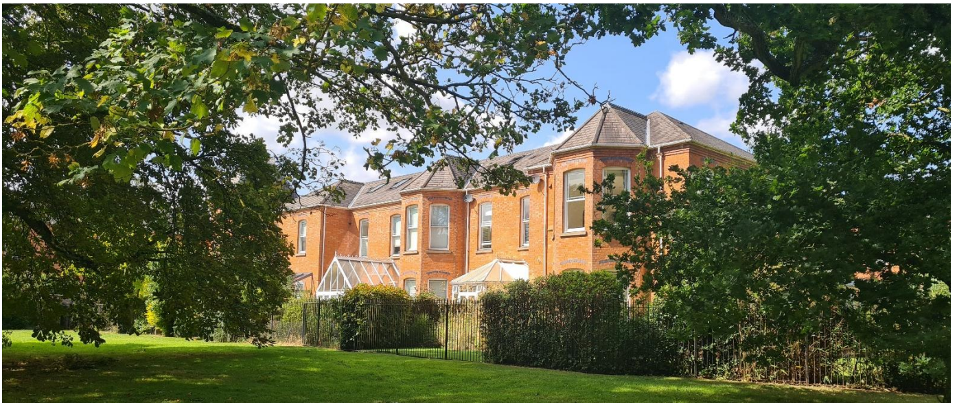
Figure 30 - The architecture of the ward buildings includes slender sash windows with ashlar sills and arched brick lintels incorporating blue brick detailing. The roof is of Welsh slate with ridge tiles and the eaves are decorated with courses of projecting bricks.
