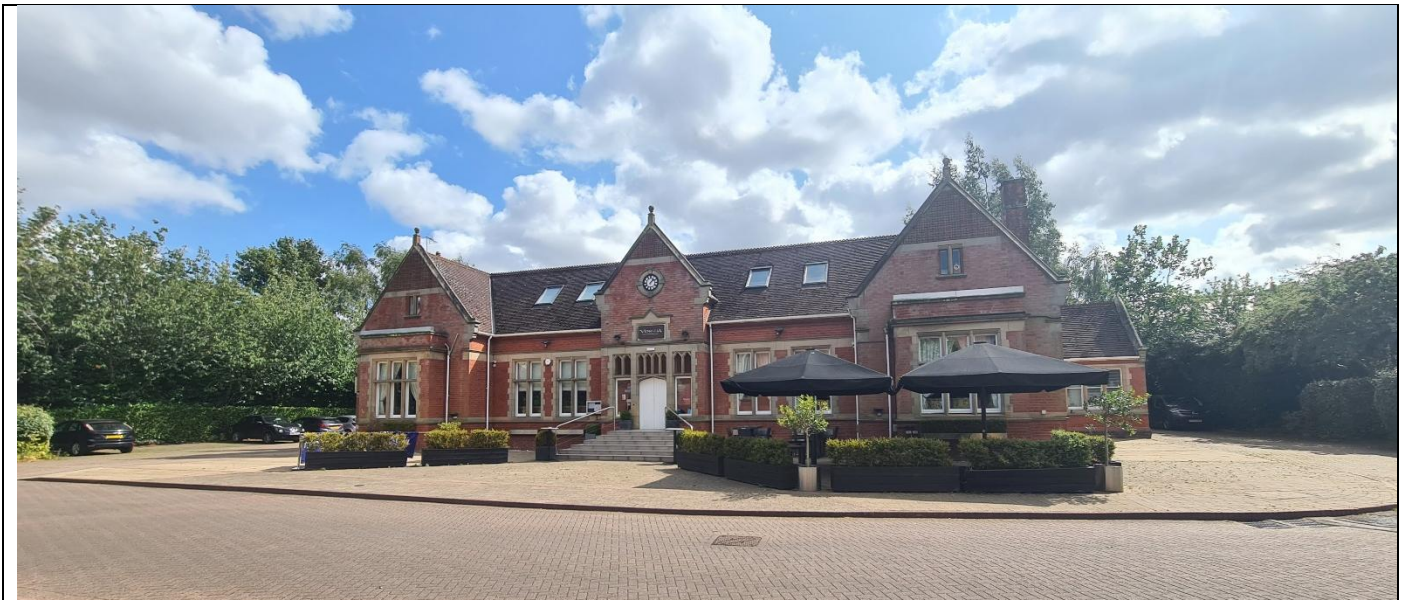
Figure 28 – The former administration building's central entrance was once the formal entrance to the hospital. The windows, door and clock face are heavily decorated with ashlar detailing. The gables are further adorned with ashlar kneelers, parapet and finial and floral terracotta diaper work. The building is now uses as a restaurant and offices.
