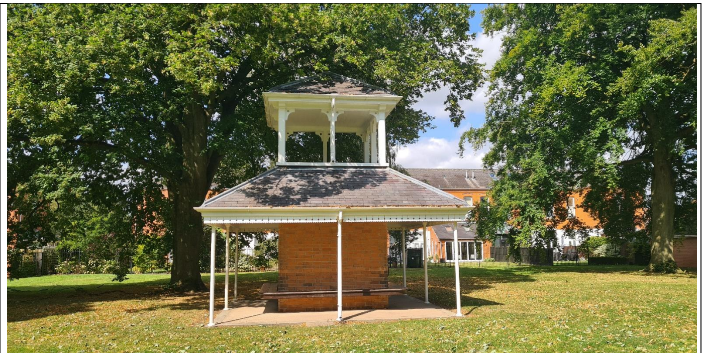
Figure 10 - one of the four garden pavilions glimpsed between the mature trees of the hospital grounds
