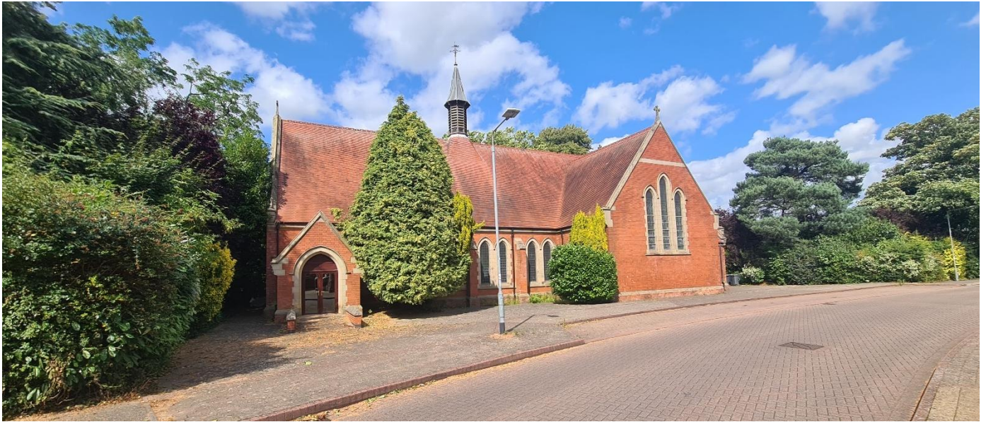
Figure 29 - The chapel has orange brick walls with ashlar door and window surrounds, kneelers, eaves lines, parapet gables and finials. The plain clay tiles cover the steeply pitched roof which is adorned with decorative ridge tiles. Openings are typically early gothic in character. The interior is finished more simply, with plastered walls and pitch pine roof. The floor is laid with maple blocks.
