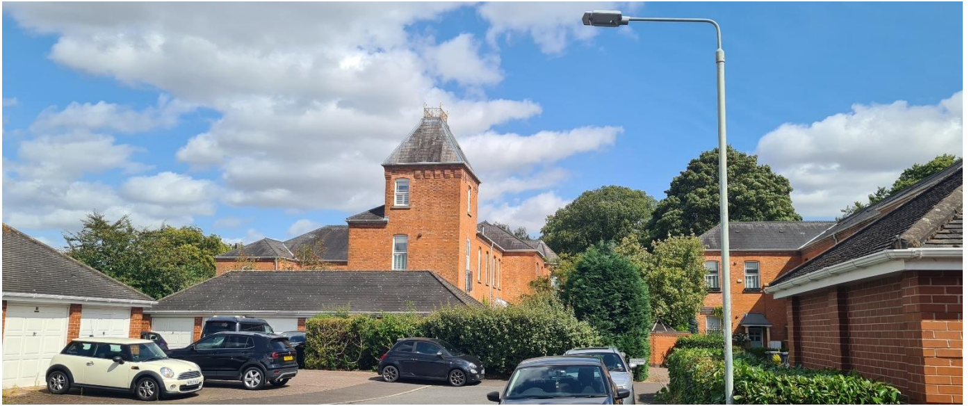
Figure 31 - One of the four towers found on the ward buildings. These have pyramidal state roofs with wrought iron finials and brick eaves detailing.
