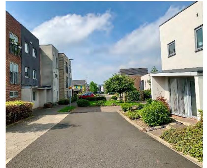
Staithe housing, Gateshead. Street designed for walking speeds. Varied planting creates a buffer between houses and street, whilst clear visibility of entrances and front windows help animate the street. (Photographs by Rob Beardsworth)
