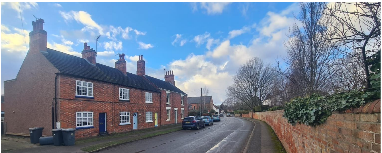
Figure 44 – Workers' cottages with Flemish bond brickwork (Zone 1)
