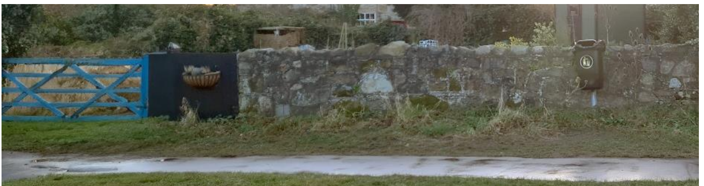
Figure 33 – Boundary stone wall at 6-8 Park Lane, (Zone 2)
