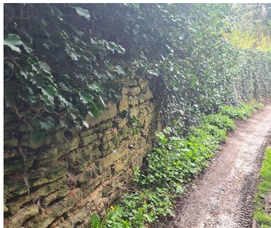
Figure 37 – Part of the stone wall visible through the ivy. (Zone 3)
