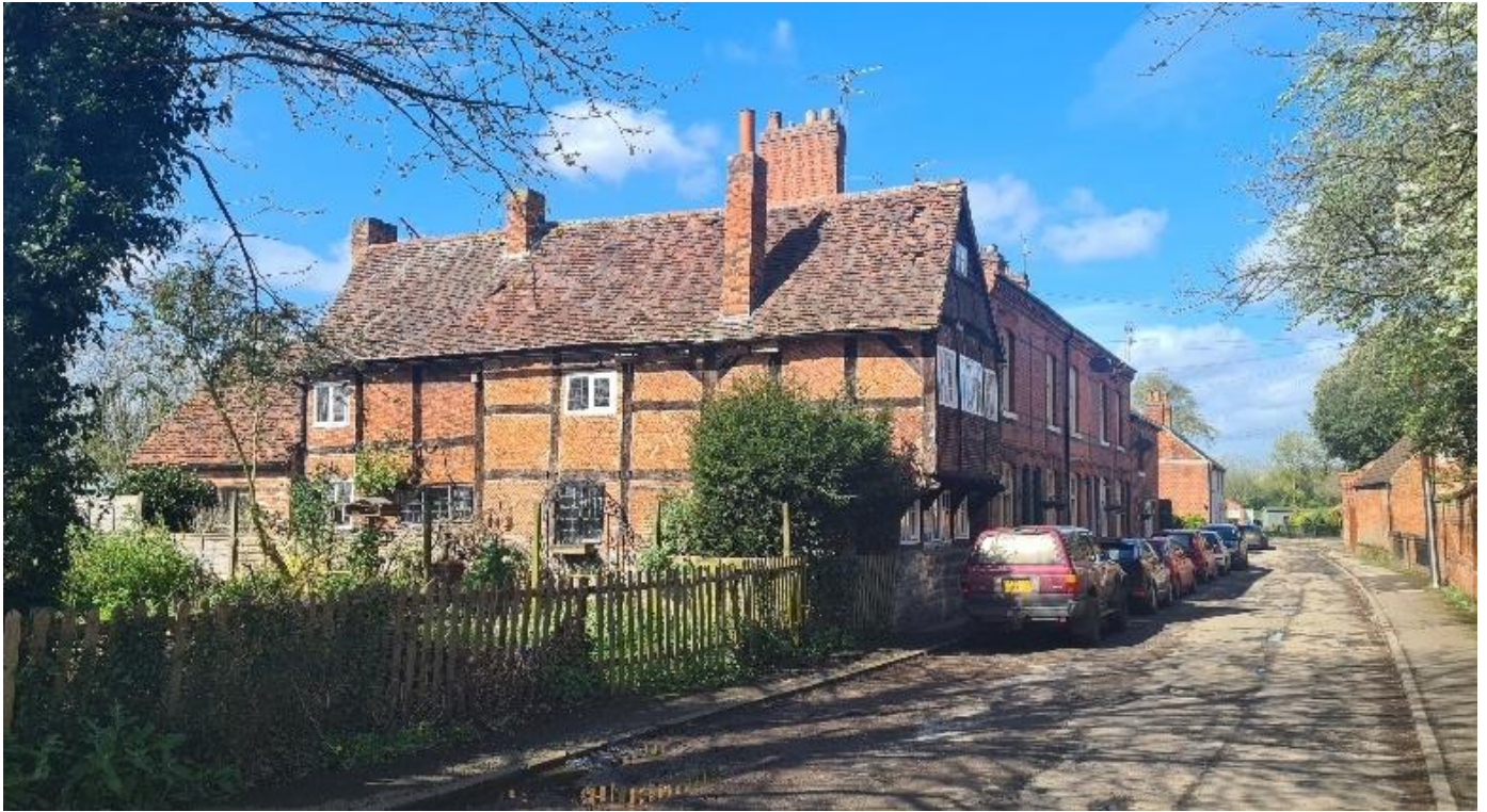
Figure 53 - Mid C17 house with C18 and C19 alterations. Timber framed with red brick nogging, in the main herringbone (Zone 1)
