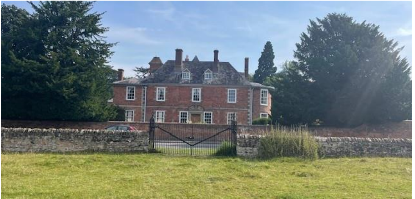
Figure 43 - The Hall (No 88 Main Street) Grade II* Small country house. Early C18 with late C18 and C19 alterations and additions. (Photo submitted by the Parish Council – a view from private land) (Zone 3)
