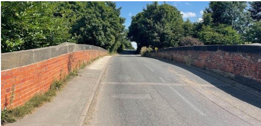
Figure 31 - Bridge Walls along Marle Pit Hill
