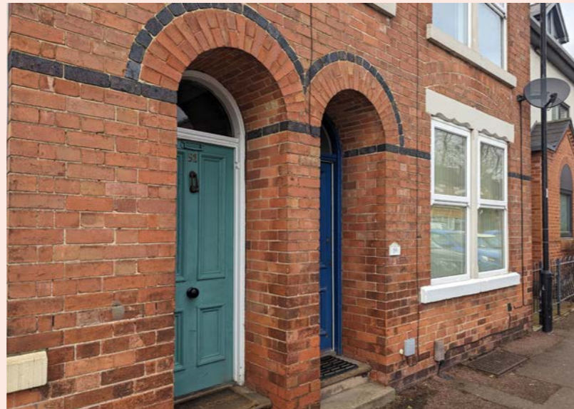
Fig 33: Paired vaulted door entrances
