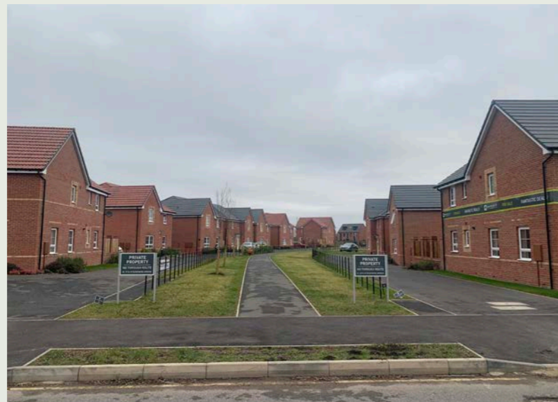
Fig 73: Pedestrian routes segregated from private drives
