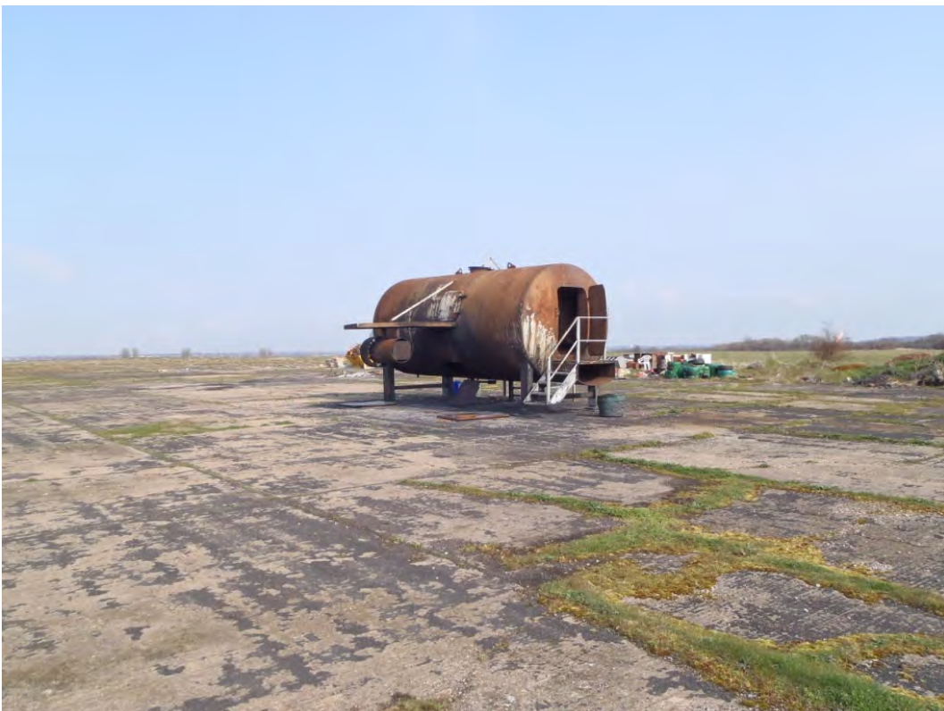
Photo 8— Fire training area.
