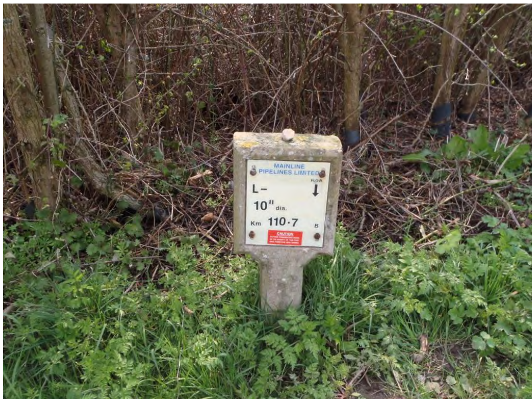
Photo 20— High pressure oil pipeline sign.
