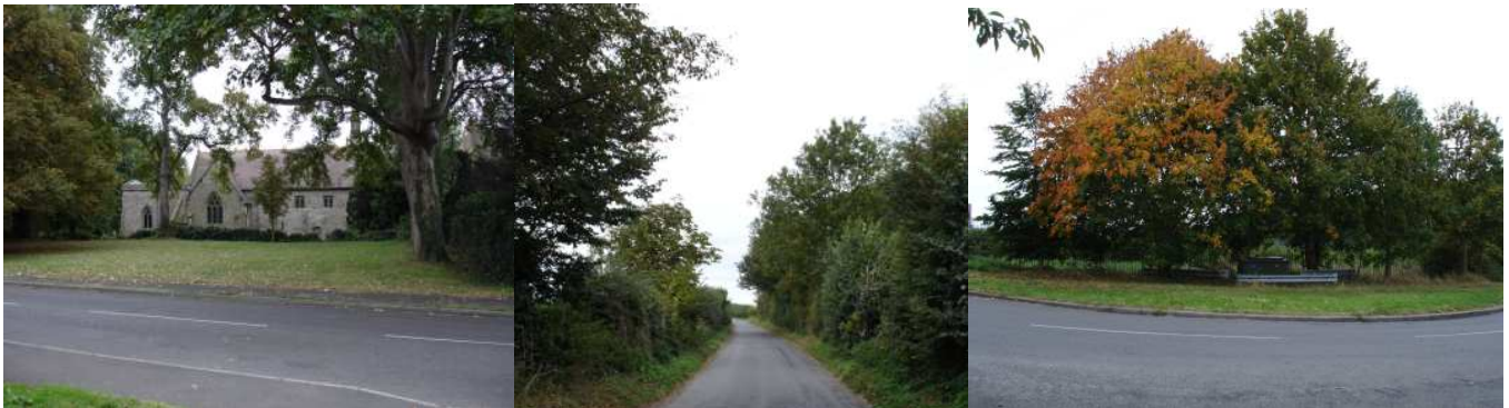
Above, left: open space in front of St Helena's Church; centre: trees and hedges along Dark Lane, right: open space and trees at the junction of Pithouse Lane and Main Street
