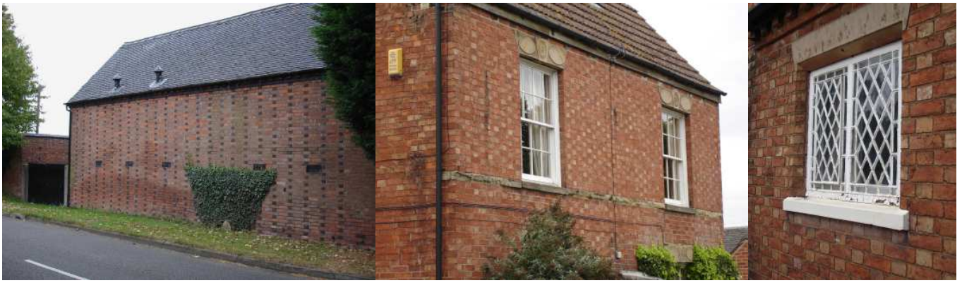
Above, left: Industrial blackened brick header detail to a barn fronting Main Street; centre: traditional timber vertical sliding sash windows on house on Main Street; right: diamond lattice metal window and Flemish bond with lighter coloured headers on the Village Hall.
