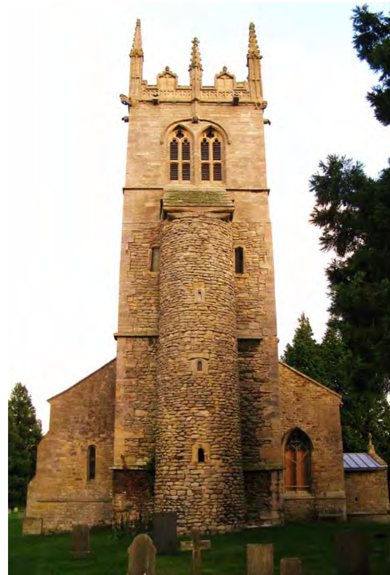
All Saints Church Hough on the Hill is Grade I listed and built of ironstone and limestone. The stair turret and lower tower are 11th century; the upper tower is 15th century.
