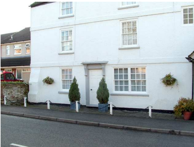
The White House: Rendered and painted walls with string courses at floor levels, Georgian style timber sliding sash windows with stone sills and a panelled timber door with decorative stone surround.
