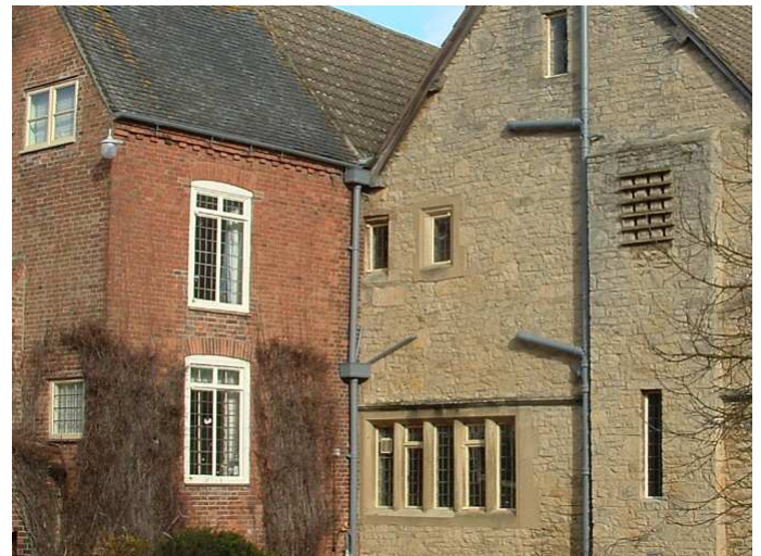
Hall Farmhouse: 17 th century rubble stone walls with stone mullioned windows and a dovecote alongside an 18 th century brick extension with larger timber casement windows, arched brick lintels, corbelled eaves and plain tile roof.
