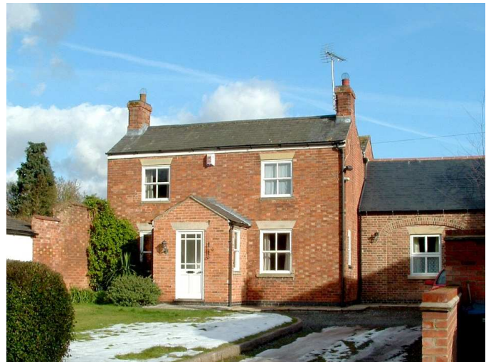
6 Chapel Lane: Chequered Flemish bond brickwork, timber sliding sash windows with stone sills and lintels, slate roofs and part glazed timber door.
