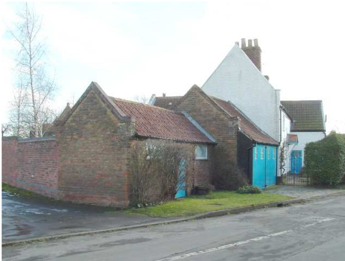
Cherry Tree Farm: Brick walled barns with parapet gables and pantiled roofs. The farmhouse has rendered white painted walls.
