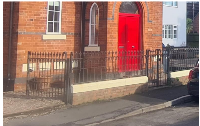
Figure 15 - Iron gates and railings on a dwarf wall
