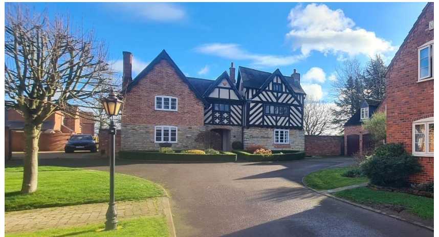
Figure 8 – The Manor House. C16 th Timber frame Manor House Farmhouse. Rubble, render, red brick, some ashlar. (Manor House Drive)
