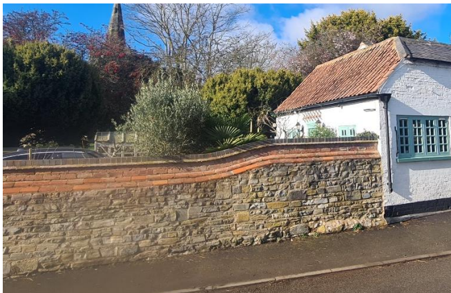
Figure 14– Stone wall with additional courses of brick
