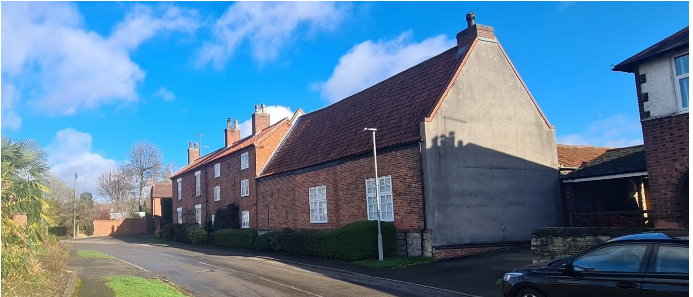
Figure 29 – A traditional farmhouse with attached barn (Pear Tree Farm, Wymeswold Road)
