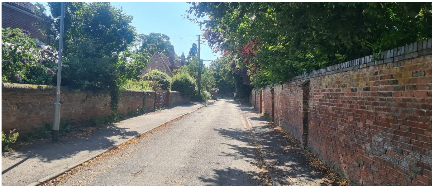
Figure 17 – Boundary Wall to Langar House and other properties along Church Lane (Zone 1)
