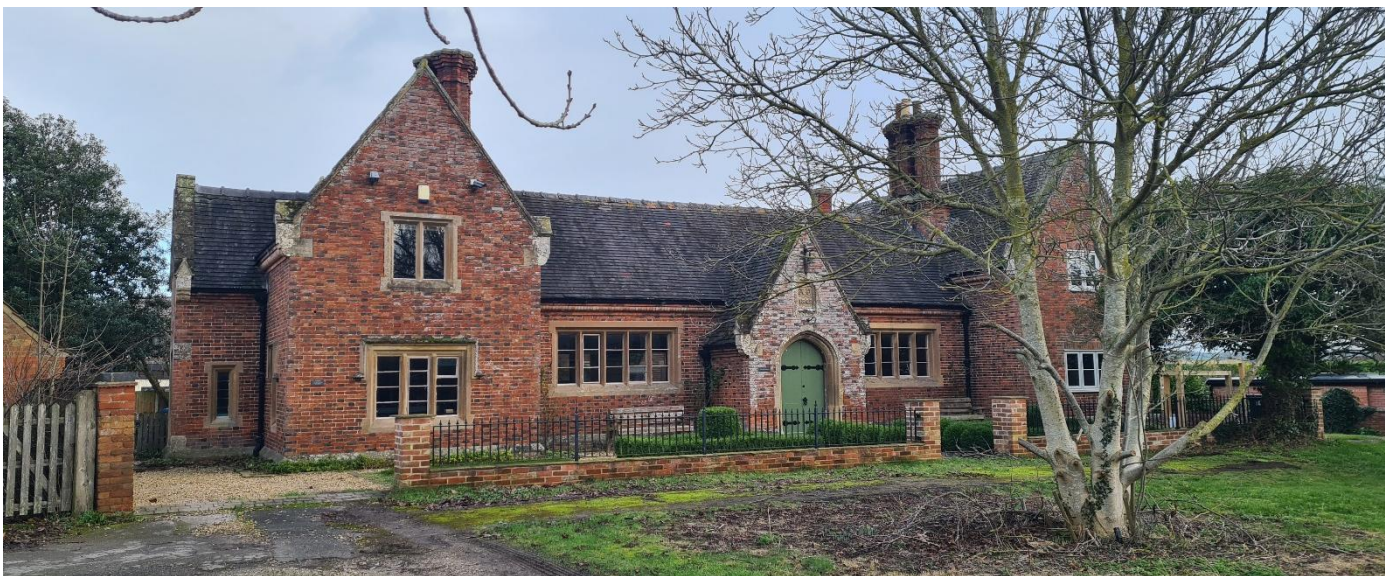
Figure 22 – Former Langar C of E Junior School and School House (Zone 1)
