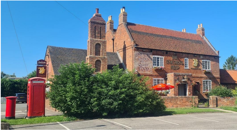
Figure 11 – The Unicorn's Head with the K6, cast-iron telephone kiosk, dating from 1935
