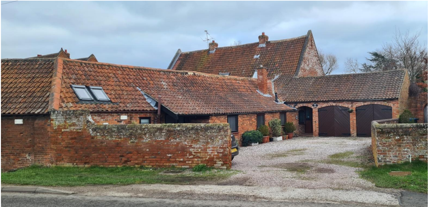
Figure 21 - Former Stable Range Immediately North of Bottom House Farmhouse including Garage to North (Zone 4)
