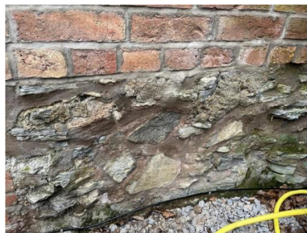
Figure 26 - C19 Brick on older stone foundations
