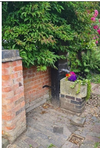
Figure 30 - Old Water Pump, 17, Church Lane
