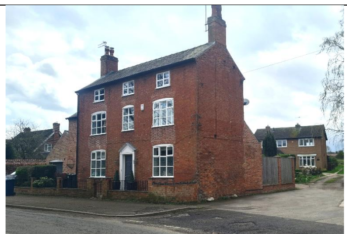
Figure 25 – No. 31, Main Street
