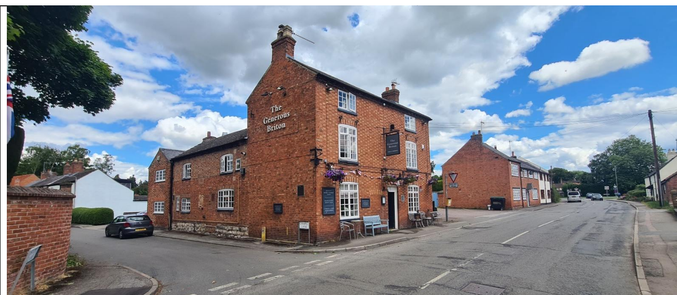
Figure 10 - The Generous Briton Public House, showing stone section along Chapel Lane
