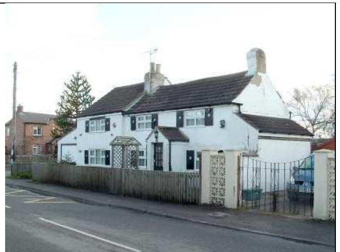
Figure 28 - No. 61 Main Street
