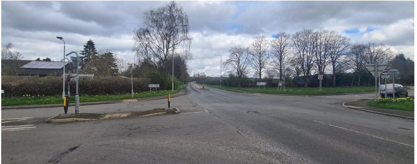
Figure 5 – Loughborough Road (A60)
