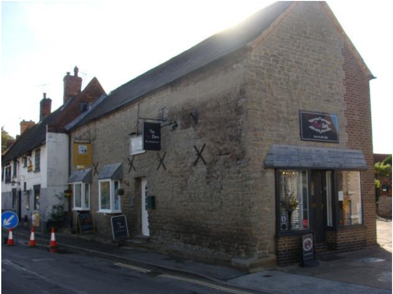
Stone buildings, particularly stone agricultural buildings, are rarities in Rushcliffe but this prominent example can be seen on Main Street at the west end of The Wheatsheaf.
