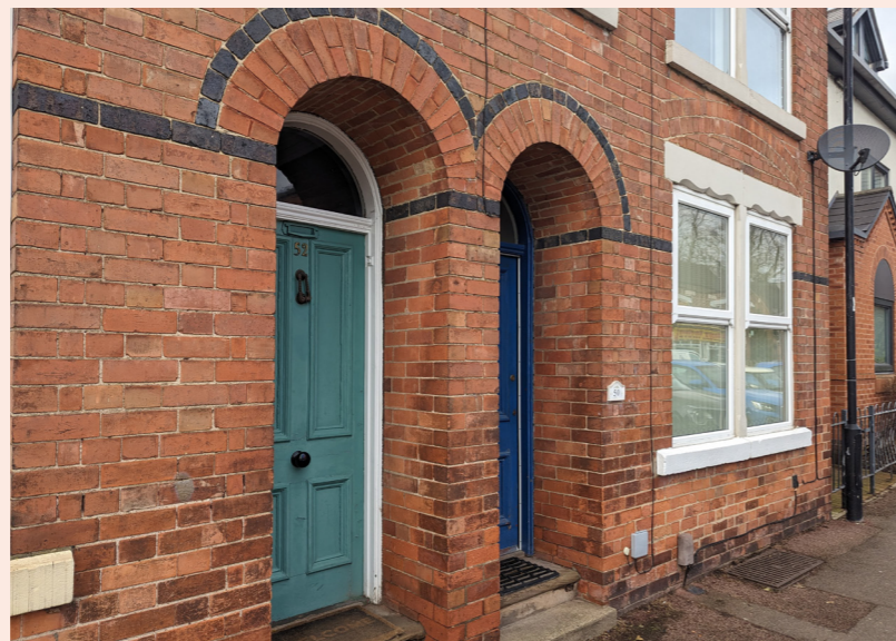
Fig 33: Paired vaulted door entrances
