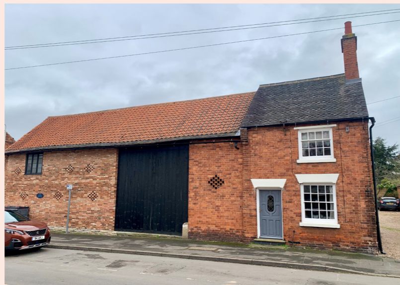
Fig 40: Barn on Main Street
