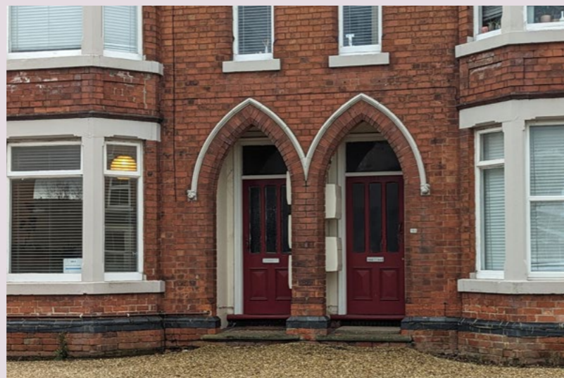
Fig 21: Distinctive bays and pairs of doors can be found throughout with arched bays displaying bespoke brick and clay work.
