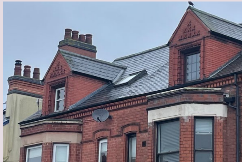
Fig 20: Motifs and ornate clay brickwork provide relief and help to define a local architectural language
