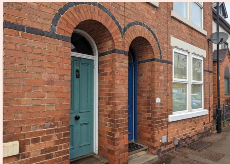
Fig 33: Paired vaulted door entrances
