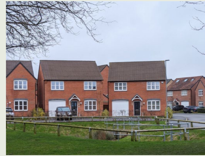
Fig 78: Detention ponds feature heavily at site entrances. Poor integration of SuDS and low value contributions to public space
