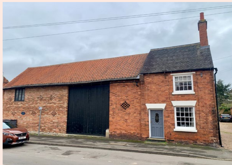
Fig 40: Barn on Main Street
