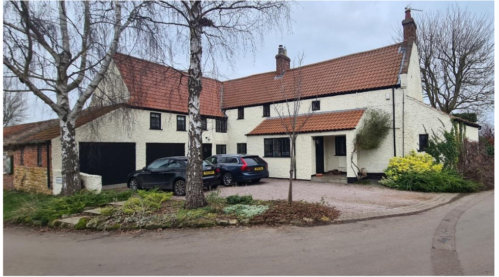
Figure 20 - Tyler's Cottage, Sunbeam Street, (Zone 1)
