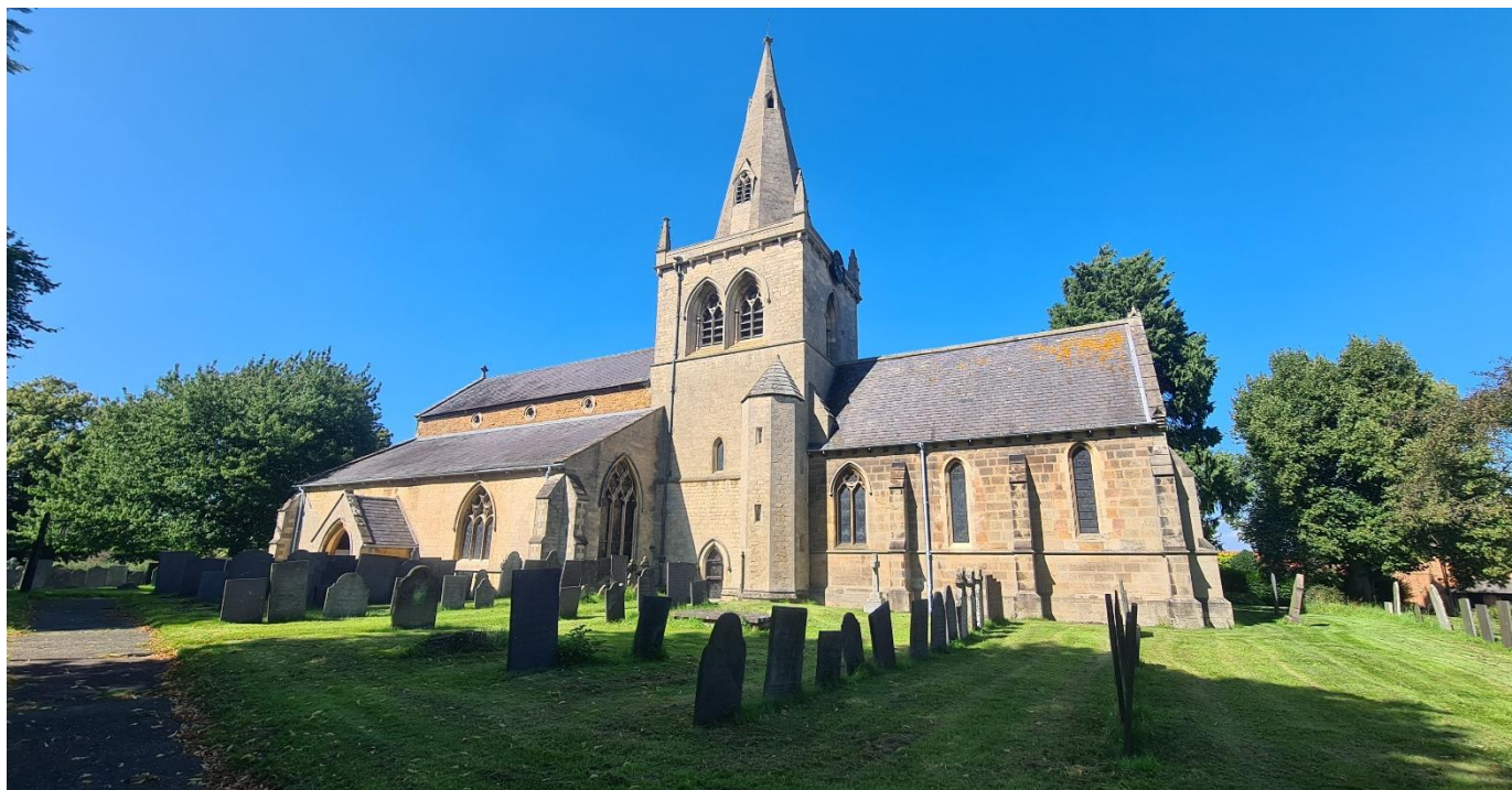
Figure 5 – St John of Beverley Church, (Zone 1)
