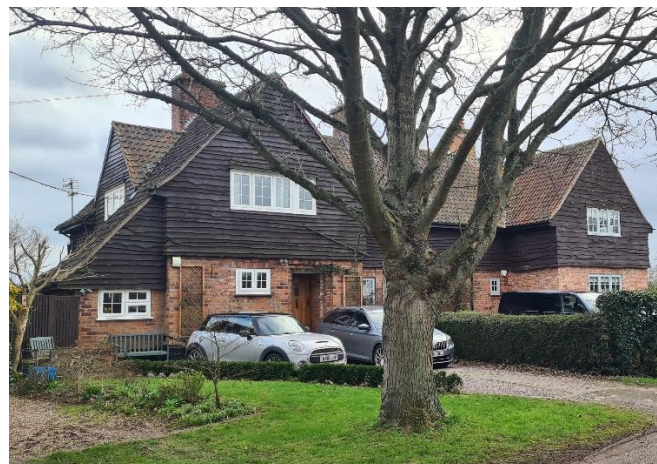
Figure 34 – Timber Cladding at 5 and 7 Conery Lane, (Zone 1)
