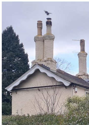
Figure 30 – Barge Board and Chimney at Elmcote, School Lane, (Zone 1)
