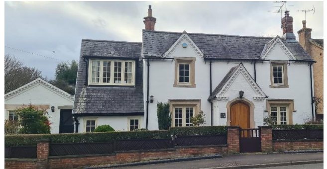
Figure 26 – The Forge, Conery Lane, (Zone 2)
