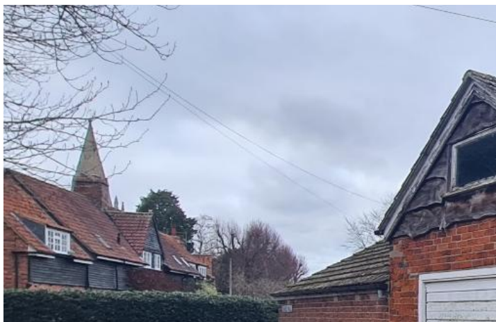
Figure 33 – Timber Cladding at Penrose, 4 Burton Lane and Chapel Walk, (Zone 1)
