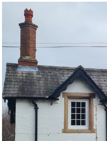
Figure 31 – Barge Boards and Chimney Stack at The Forge, Conery Lane, (Zone 2)
