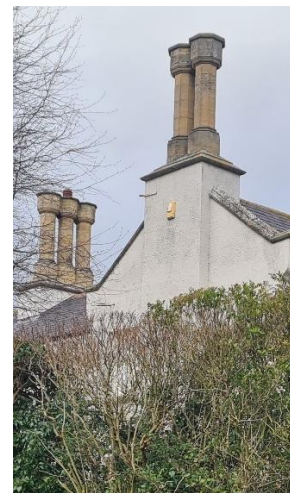
Figure 32 – Chimney Stack at Whatton House, Conery Lane, (Zone 2)
