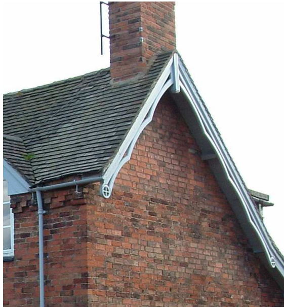
Carved timber barge boards and plain tile roof (Elton Cottage).
