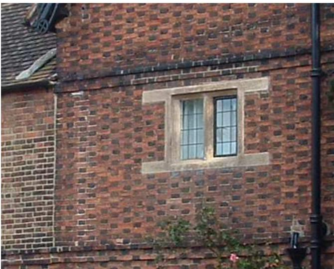
Chequered brickwork, decorative string courses and stone mullioned casement window with square lattice (Church House).
