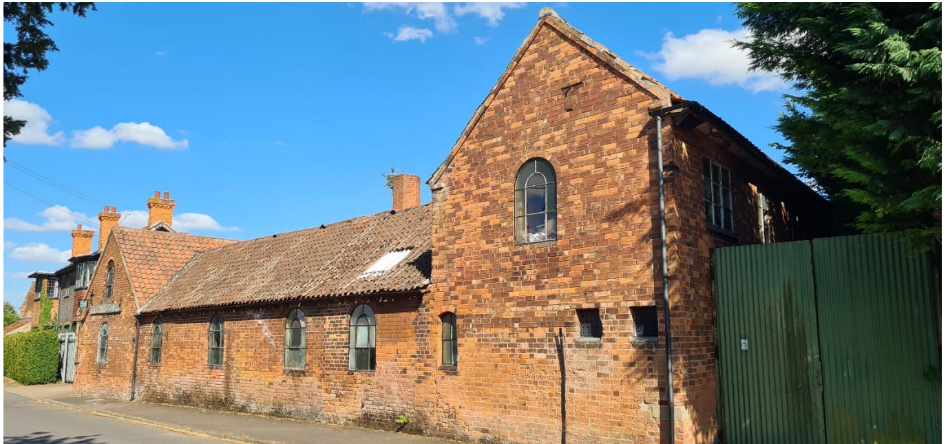
Figure 21 - Progress Works, Main Road
