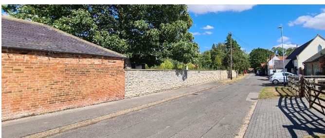
Figure 16 – Hawksworth Place Garden Wall to Town Street and Top Farm Fence and Gate
