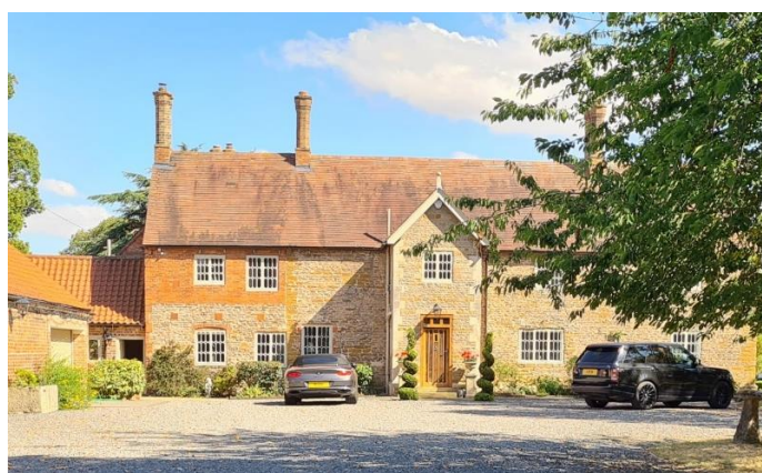
Figure 23 - Hawskworth Manor and Adjoining Pigeoncote (Grade II)
