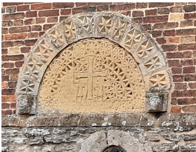
Figure 3 - Tympanum on the South Facade of the Church
