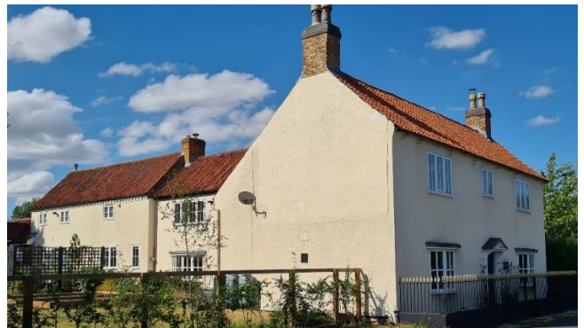
Figure 32 - Ivy House Farm (Main Road)
