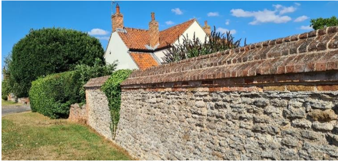
Figure 18 - Hawksworth Place Garden Wall to Main Road
