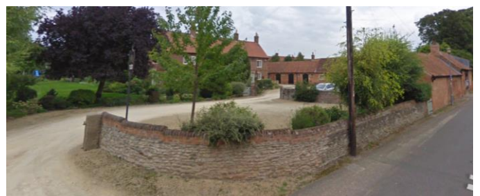
Figure 17 - Yew Tree Farmhouse Garden Wall with Partial Rubble Plinth
