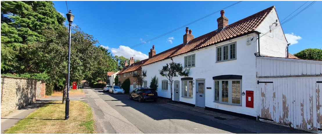
Figure 12 – Town Street towards Hawksworth Manor
